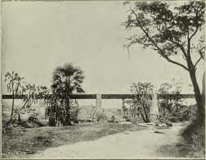
THE COMPLETED TSAVO BRIDGE.
